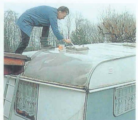
Sheet metal roofs of all kinds: seal leaky areas.
