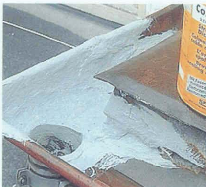
Repair gutters permanently, simply by brushing on.
